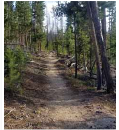
Bike trail corridor cleared to specs Photo: NPS
