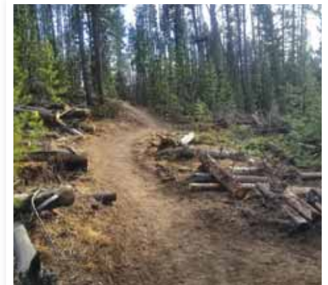
Grade reversals were constructed to minimize erosion. Photo: NPS
