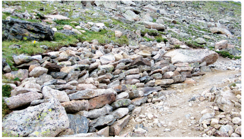
New rock wall supporting the tundra and preventing erosion on the Longs Peak Trail
