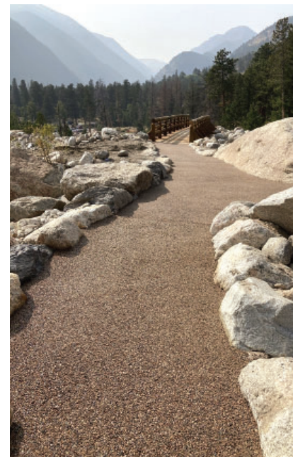
Finished paved trail near the Alluvial Fan Bridge
