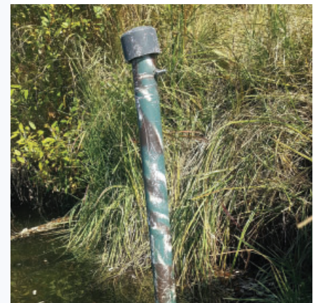
Water monitoring well and stream gauge that document changes in water levels near the simulated beaver structures.
