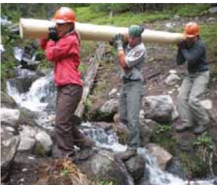
2018 Boulder crew building bridges
